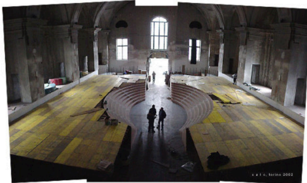
the arena under construction
